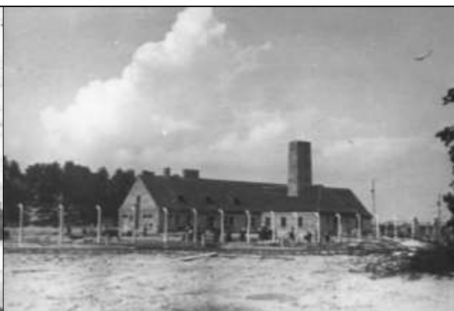
The finished Crematorium III.
